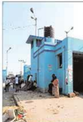
The subway near the Calcutta bus stand is cleared giving free way to commuters
