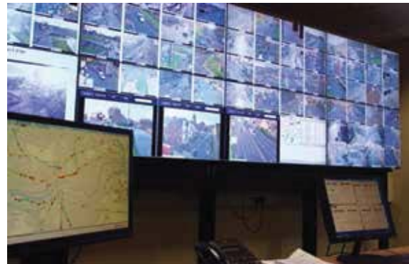
Fig. 4.1: Traffic Management Centre at Newcastle University
